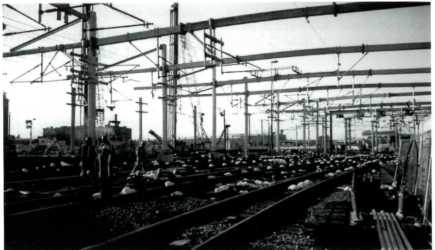
Figure 2. The Big Freeze - Artificial ground freezing in the track area near Boston South Station
