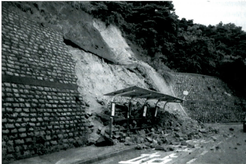
Figure 1. Near ground surface, engineered structures, such as this protected slope in Hong Kong, become unstable in response to extreme changes in moisture flux boundary conditions.
